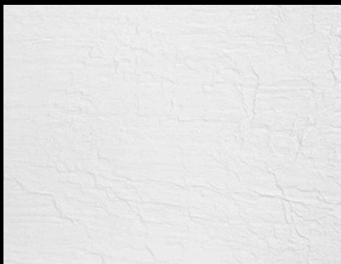
Soft Stone Surface Width: 4' (48 in) Height: 8' (96 in) BH-R-1
