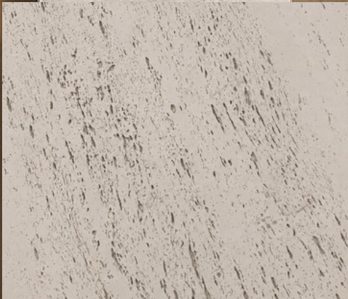
Soft Stone Surface Width: 2' (24 in) Height: 4' (48 in) BH-R-10
